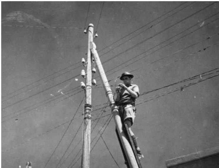
A member of a signals unit repairing telephone lines after a strafe by the Germans
